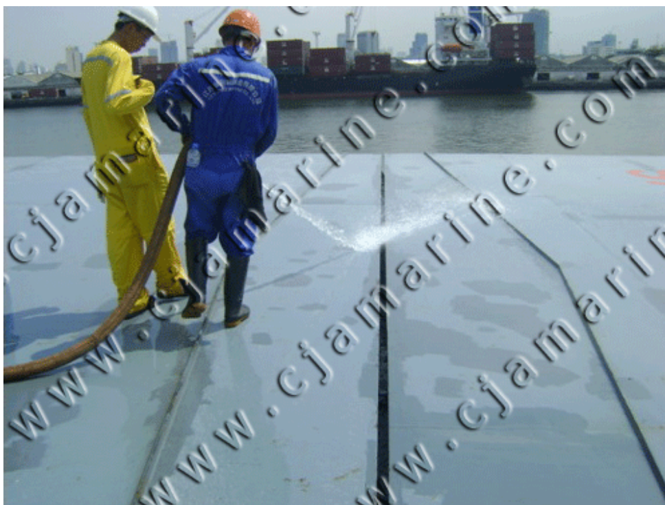
Hose Test on Hatches
